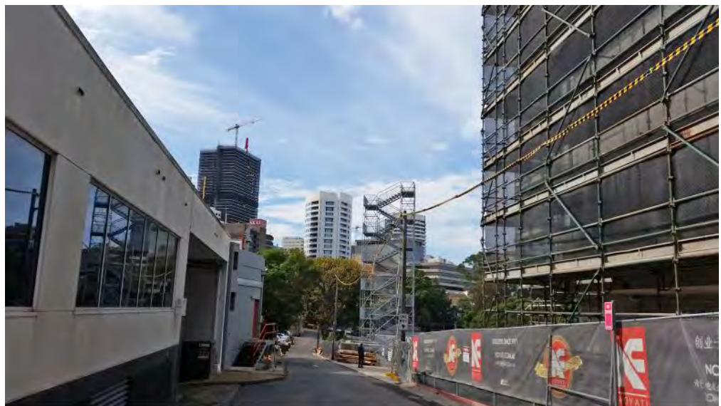
Figure 3 Marshall Lane street frontage (looking east)
