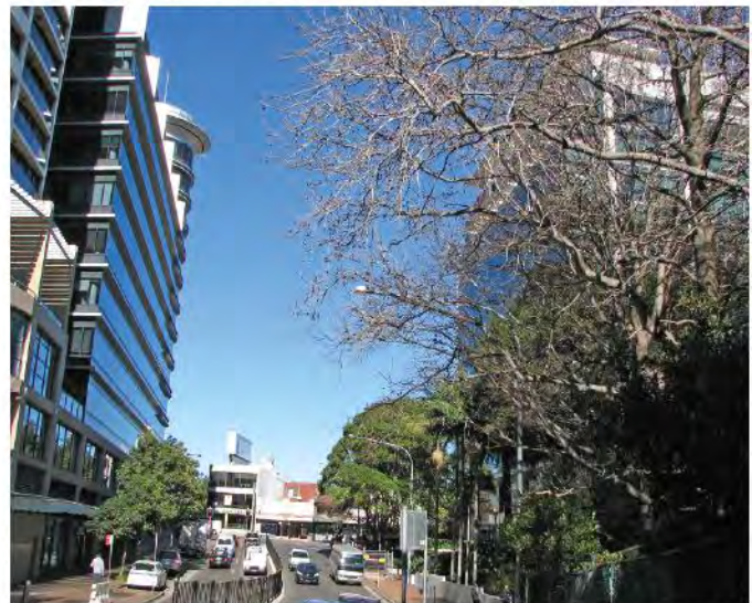
Photo 6: View south along Herbert St (tower will terminate the vista)
